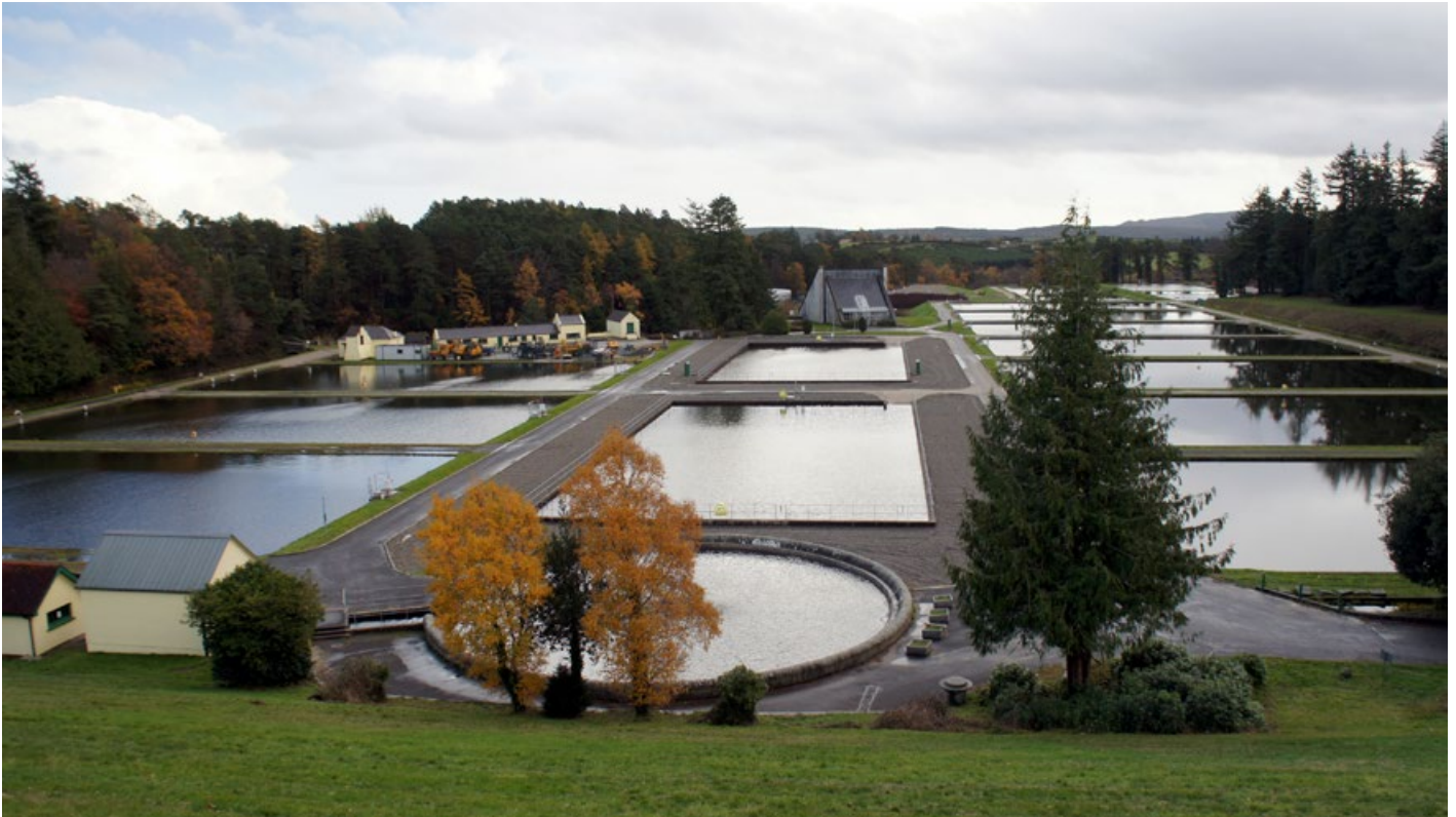
Water treatment facilities at Vartry Reservoir.
